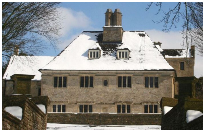
Rudloe Manor, allegedly built (or, more probably, substantially rebuilt) by Thomas Goddard Snr. in 1685. This building is on the Heritage at Risk register maintained by Historic England, and it is highly regrettable that such a fine building has been allowed to fall into disrepair. (Photo Carol Payne)
