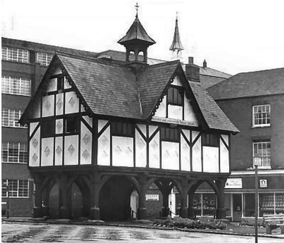
Market Harborough Old Grammar School is close to the site of the Harborough Bank
