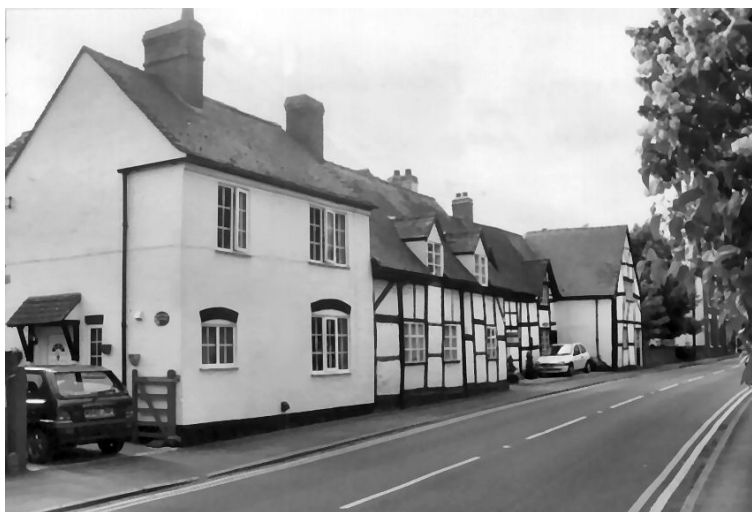
Eckington main street,-the Tewkesbury to Pershore road
